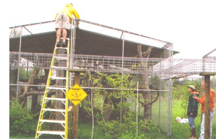
Mircio Moretti on ladder installing rain equipment
